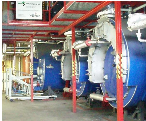
Obr. 18: Kotelna na biomasu [14]
