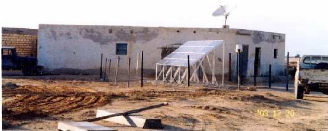
Figure 2-14: PV isolated system in countryside.
