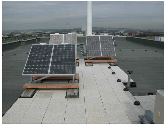
Fig. 3: PV modules with the different angles
