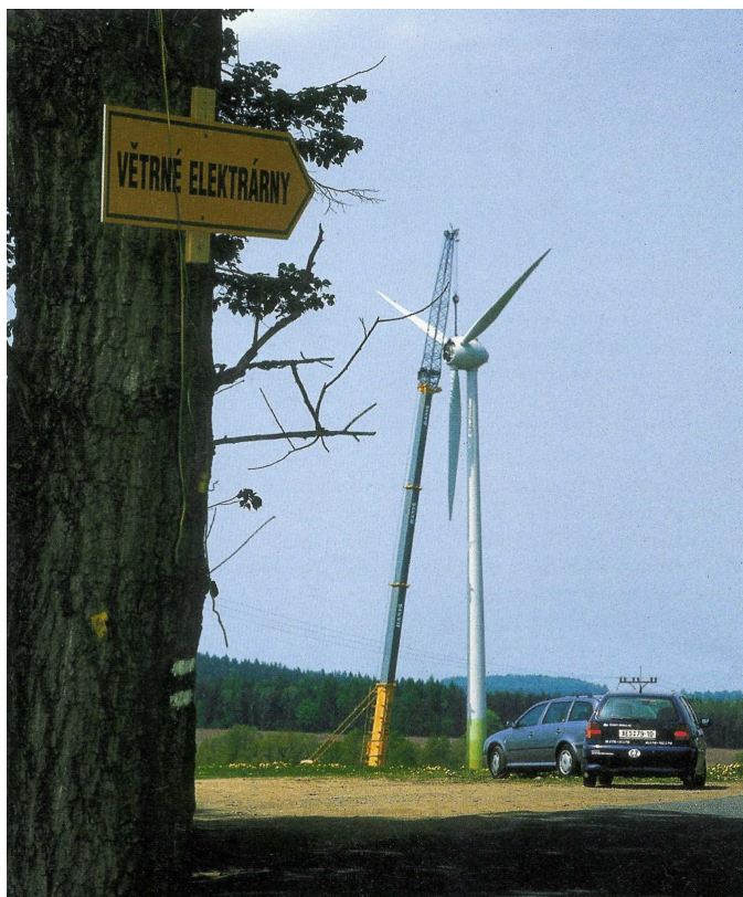
Fig. 1 – The wind power plant in the Czech Republic (photo from 2005)
