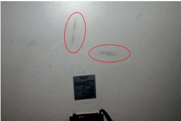
Fig. 3. PV panel damage after close lightning strike.
