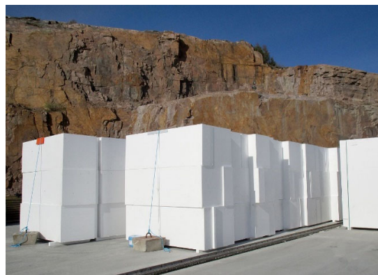
Figure 1-2: EPS geofoam blocks at a construction site
