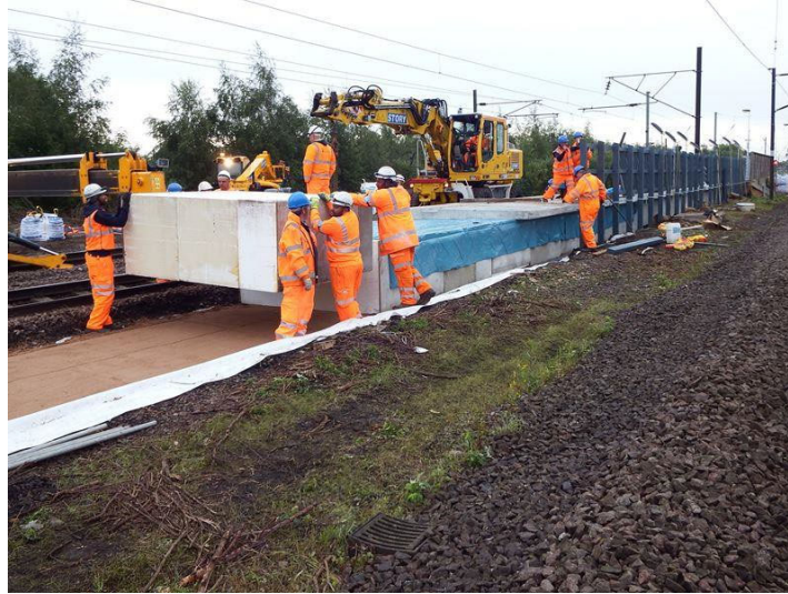
Figure 1-15: Installation of a replacement platform, similar to that at Watford, using geofoam
