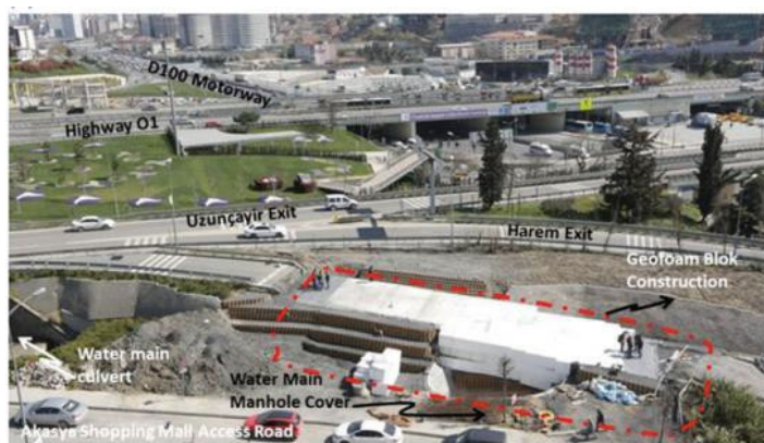
Figure 1-14: Construction area of the EPS geofoam embankment [17]
