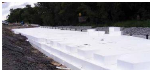
Figure 1-7: Borman Expressway (Gary, Indiana) reconstruction using EPS geofoam fill [4]
