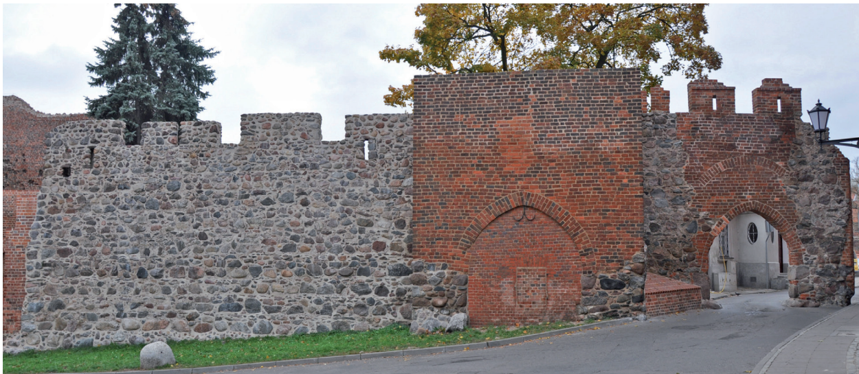
Fig. 8. Toruń. Stone wall from the middle of the 13 th century. Photo B. Wasik.
