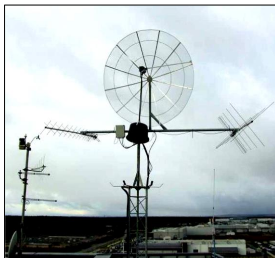
Figure 10. The antenna system of Pilsen's GS, located at the University of West Bohemia.
