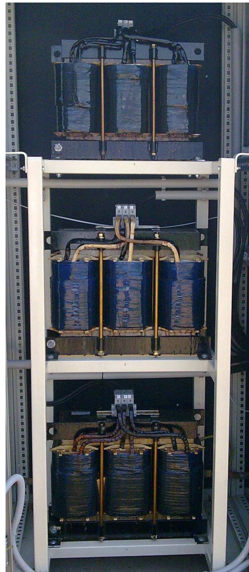
Fig. 4: Practical realization of compensation unit for PVE
