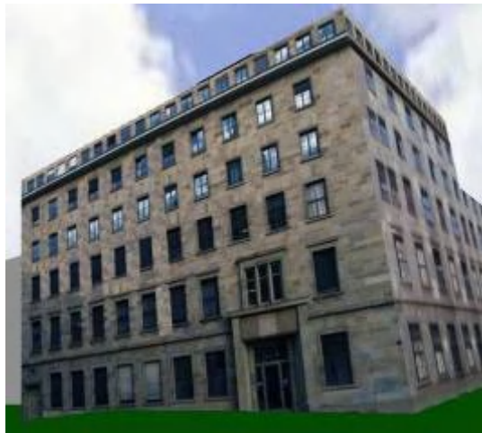
Figure 1: Mapping the images after rectification, obstacles removal and radiometric adjustment on the light weight geometry of Building 2” of Stuttgart University of Applied Science in VRML 2.0
